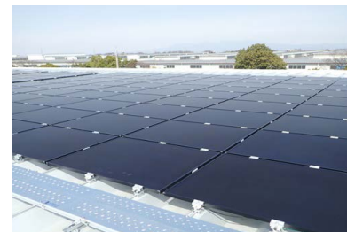
The roof of the new cafeteria
