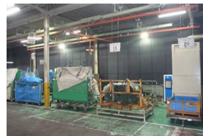
Soundproof sheets installed in the plant building
