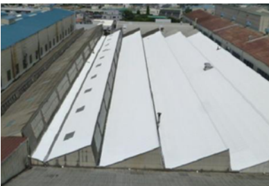
Roof with thermal barrier coating
